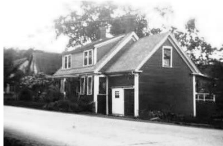
The 1834 schoolhouse is now part of a private home on Lisbon's South Main Street.
