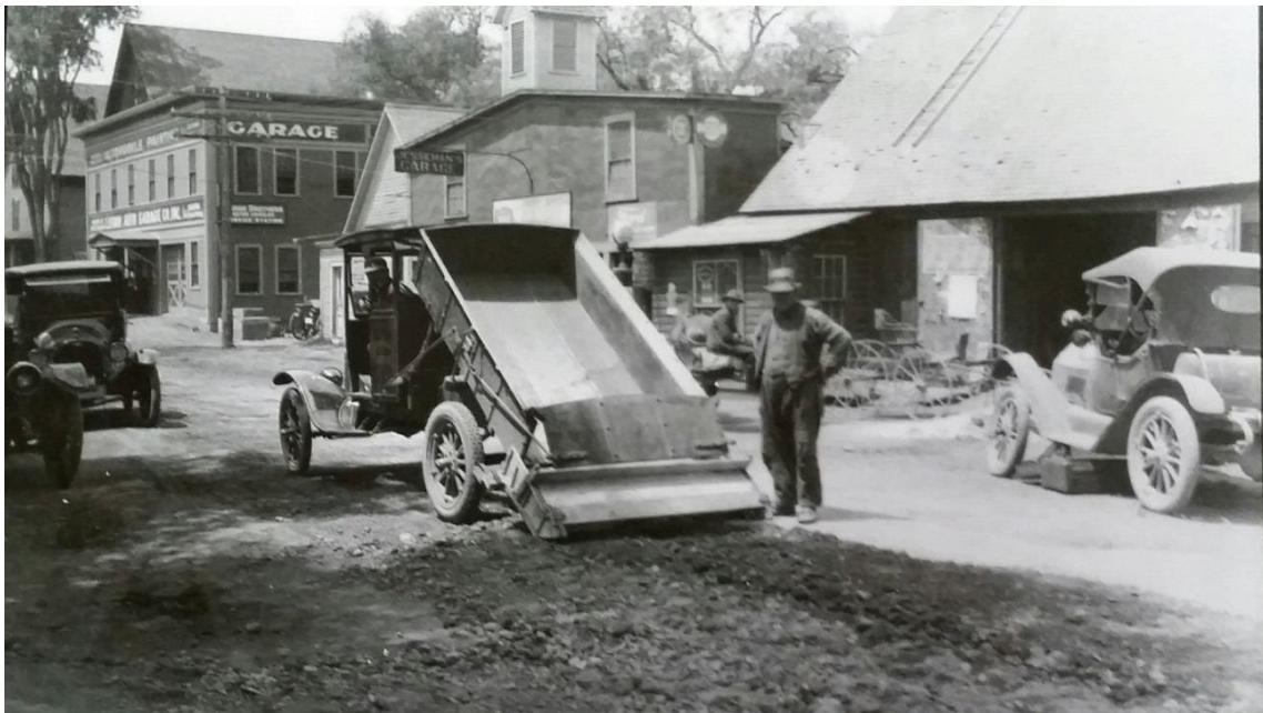
Lisbon Selectman Allen Ash stands by the town's gravel spreader on Main Street c. 1926.
