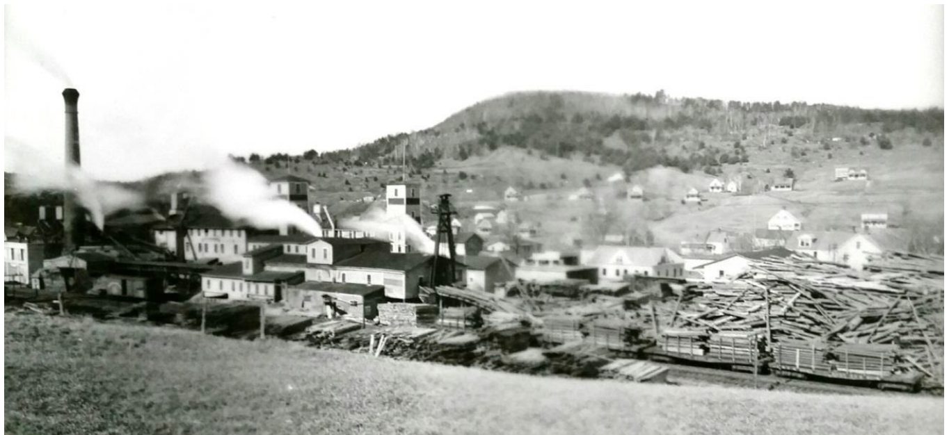
Parker Young Company on South Main Street looking east to west in its heyday going full steam with its lumber operation and manufacturing of piano sounding boards, boxes, hardwood flooring, and custom cabinetry.
