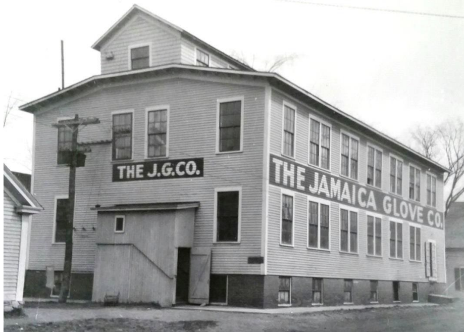
This building was originally built at the top of Whitcher Street c. 1901 as a factory for Granite State Wire, an early and unsuccessful competitor to New England Electrical Works, now New England Wire Technologies. The Jamaica Glove Company factory was in business from 1913-1934. It is now a warehouse for White Mountain Footwear.
