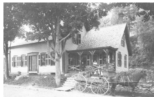
Gould home, School Street, on right before hill and sharp corner
