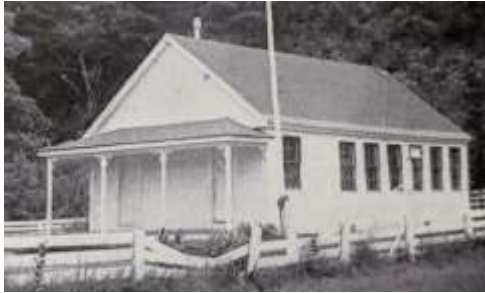
The North Lisbon one-room schoolhouse stood just before today's Varney-Smith Lumber property and was built in 1909 on land purchased for $5. It was closed in 1959.
