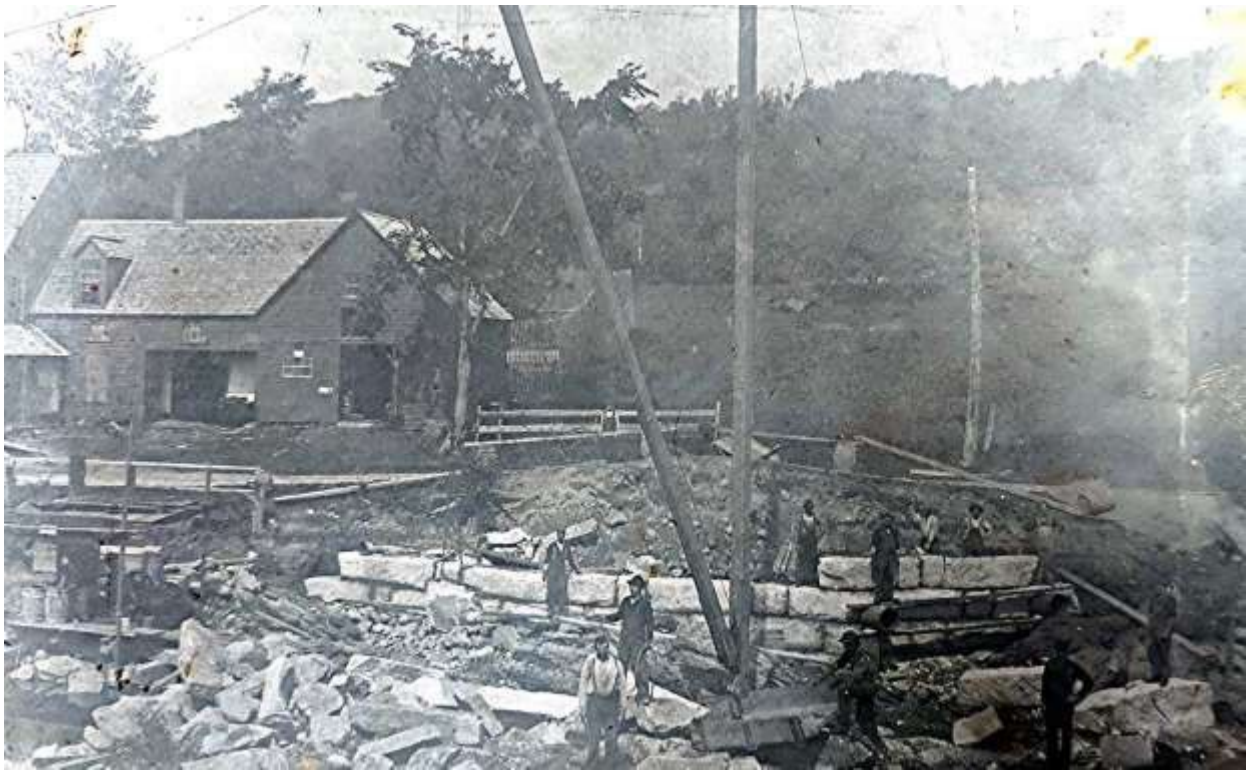
Work begins on building a new bridge at Barrett's Crossing after the flood of February 1896
