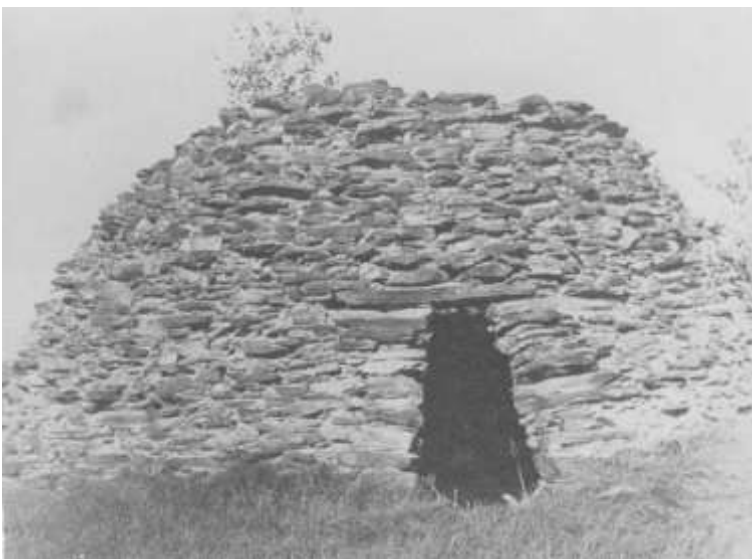
The Lisbon coal kiln c. early 1900s is pictured after its top dome stones had been removed. The original kiln was in the shape of a complete beehive.
